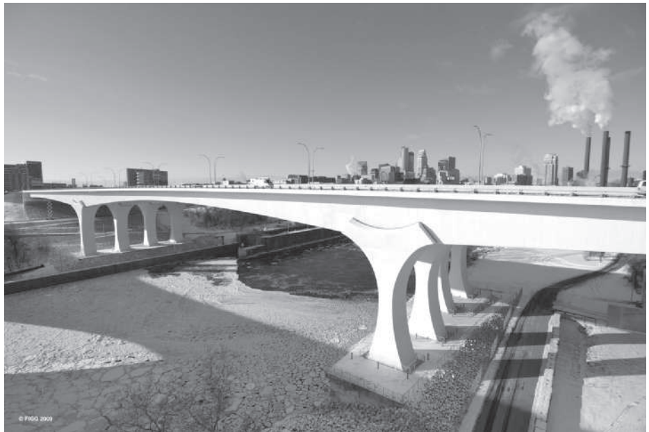
Fig. 1-3 St. Anthony Falls Bridge. (Photograph courtesy of FIGG Bridge Engineers, Inc.)
